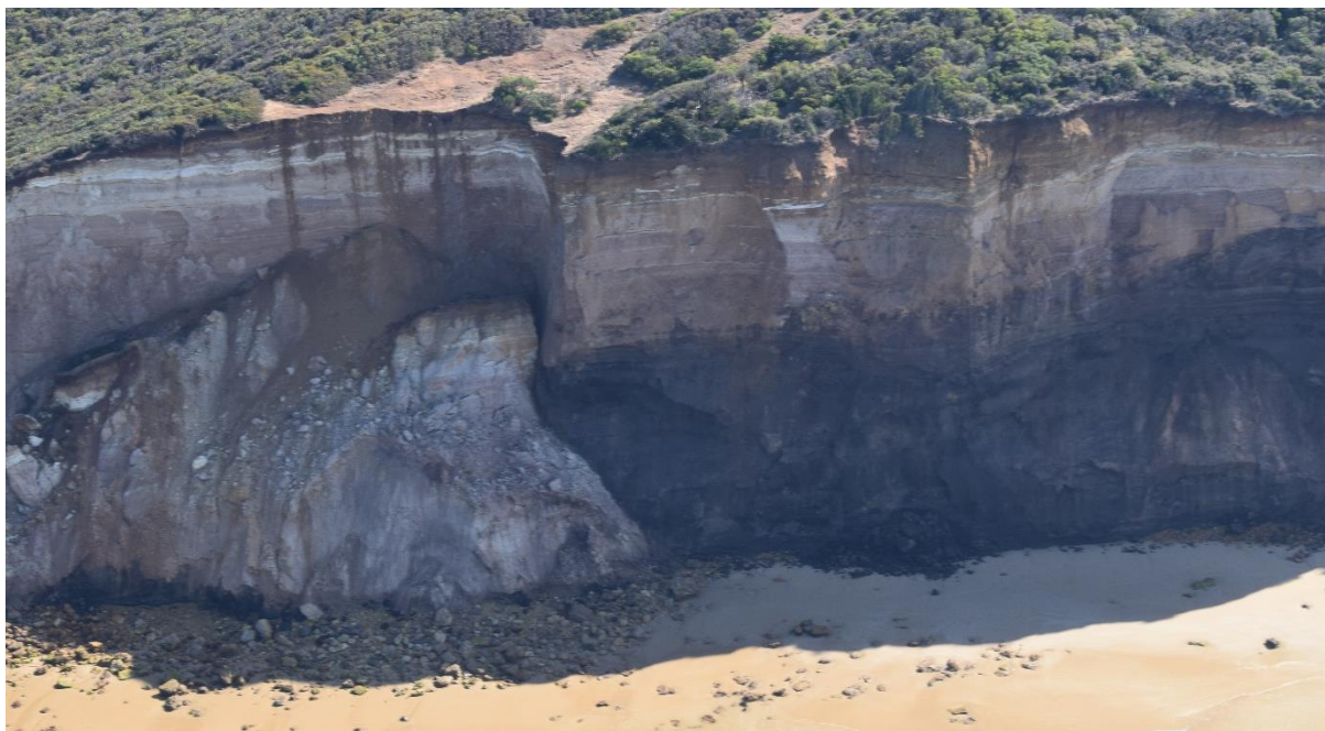
Figure 1.1: Example of cliff failure including talus runout north of Point Addis Beach (taken 24 April 2023)
