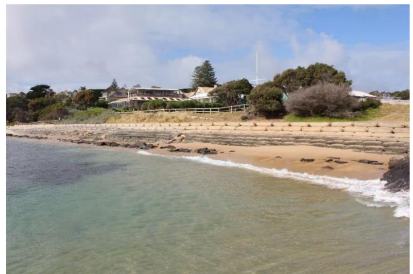
Source: Geotextile bag revetment at Portsea https://www.mornpen.vic.gov.au
