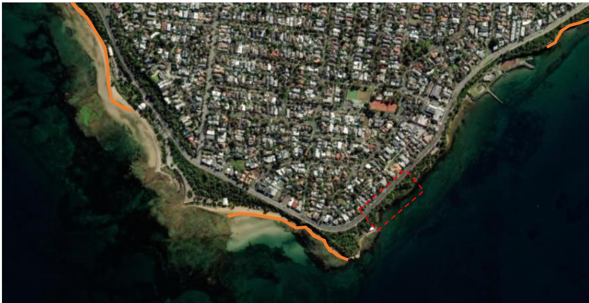
Figure 6.8: Example of a section of cliff at Beaumaris which is not included in the Water Technology Smart Line data.
