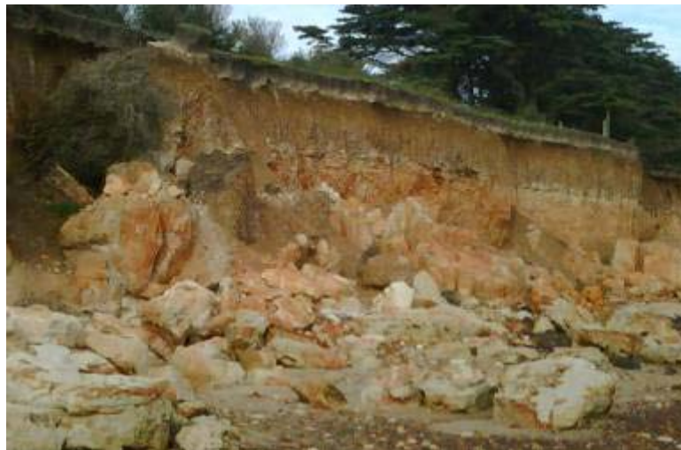
Figure 10: Active erosion at Red Bluff
