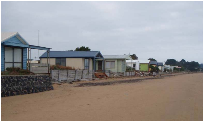
Figure 12. Boatsheds on the Lang Lang Foreshore Reserve. (Photo courtesy: GHD, 2009)
