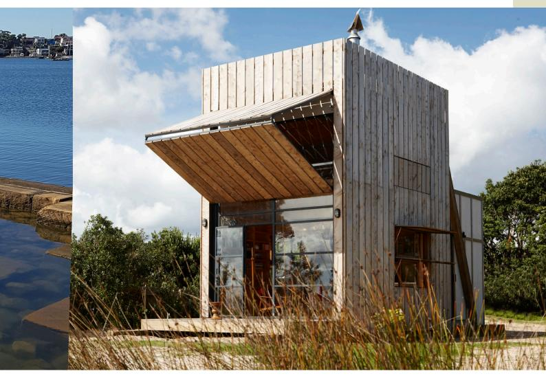
The structure is a compact building featuring sustainable water-saving waste treatment system and flexible screens. It uses ecologically friendly materials and incorporates sustainable, closed-loop systems (a worm tank system to treat waste and two tanks for grey water that can be recycled). When not in use the building is 'boarded up' and blends in amongst the dunes. (The Whanapoua Sled House, Coromandel Peninsula, New Zealand, Photo: Jackie Meiring)
