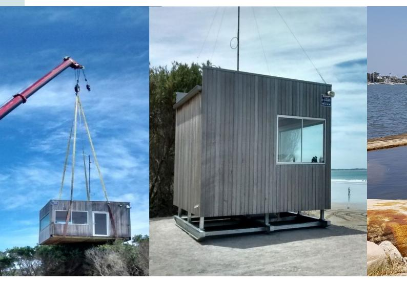
The life-saving club structure minimizes its impact on the primary dune through the setback of the clubhouse behind the dune. A low impact, modular and movable observation structure provides an alternative to hard engineering options with the ability to be moved in response to dynamic natural coastal processes. (Inverloch Surf Life Saving Club, Victoria, Photo: DELWP)
