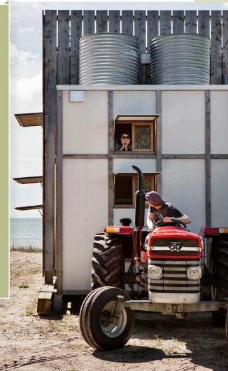
This structure incorporates innovative construction techniques to adapt to local conditions of erosion and sea level rise. The pavilion is perched on two thick wooden sleds which maximise flexibility by allowing movement around the beach as erosion or weather conditions dictate.
