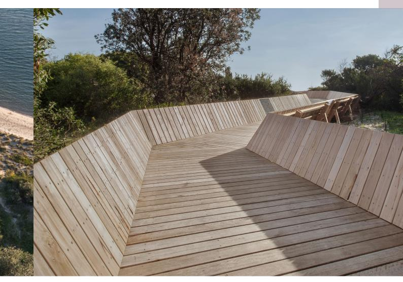
The boardwalk protects the coastal dunes from intrusion and erosion by encouraging clear and controlled movement to and from the beach. (Photo: Lisbeth Grosmann)
