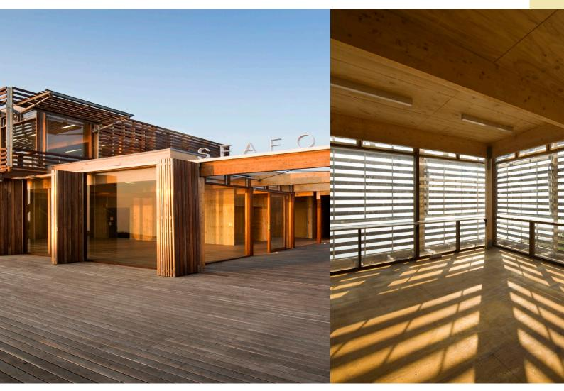
Exposure to wind and solar penetration is managed through careful orientation of building elements. (Seaford Life Saving Club, Seaford, Design: Robert Simeoni Architects, Photo: John Gollings) Timber batten screens optimize natural light and facilitate cross ventilation but can be adjusted to provide protection from prevailing winds or shield against summer sun. (Seaford Life Saving Club, Seaford, Design: Robert Simeoni Architects, Photo: John Gollings)
