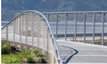
**Steel** - structural grade and hot dip galvanised as per AS/NZ 4680 for superior performance and powder coated for corrosive protection. Photo: Jarle Waehler
