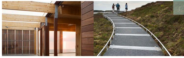
Hardwood timber - plantation - grown and recycled timber treated for protection from insects and decay - Red Gum, Jarrah and Tallowood are most durable and suitable for structure is the water. Photo: John Gollings
