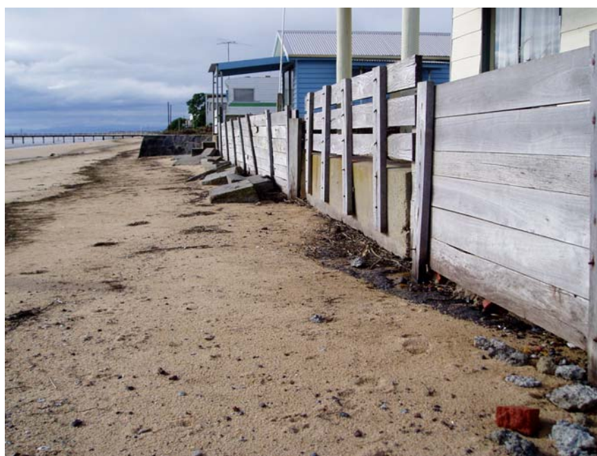
Ad-hoc, homemade seawall in front of the beach shacks
