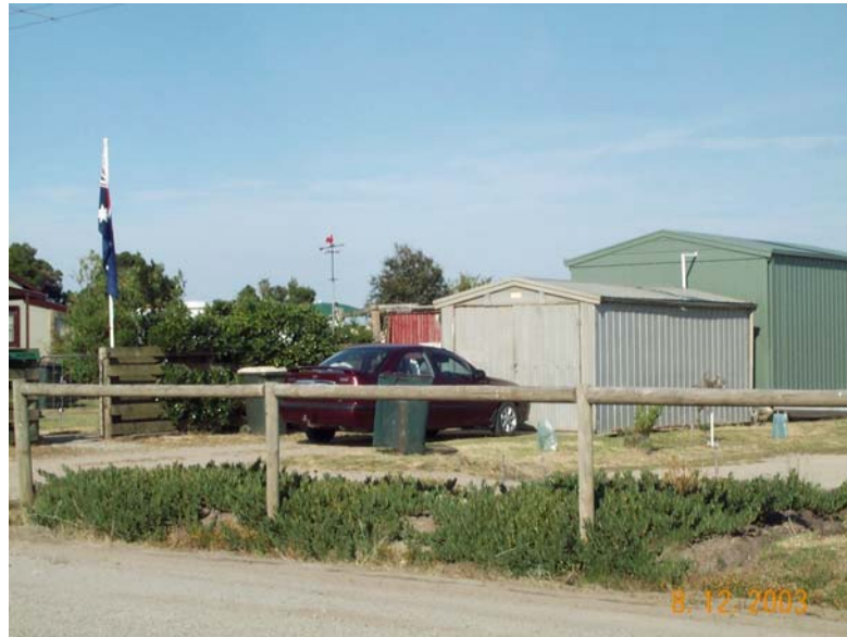
Storage sheds adjacent to caretaker's residence
