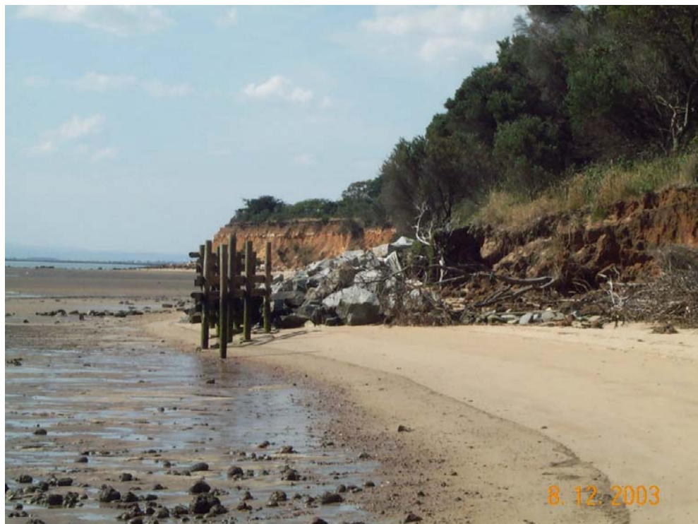
Rockwall at Jam Jerrup with terminal scour
