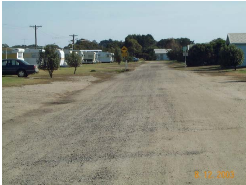
Wide gravel access road through Caravan Park
